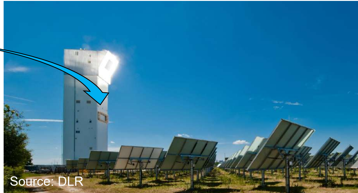
...and solar tower in Jülich, Germany
