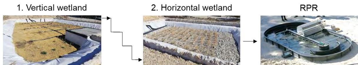
**Fig.1.** Demonstration system of natural based solutions coupled with advanced solar tertiary treatment in Murcia, Spain.
