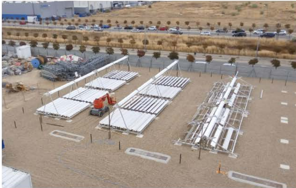
Ref: SOLATOM (Construction of Magtel project)
