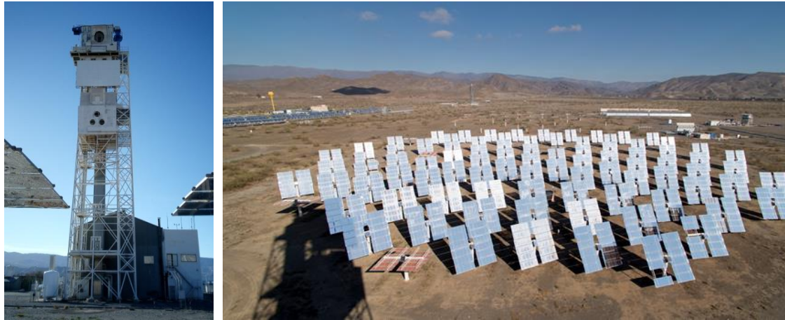
Figure 3. Central Receiver System (CRS) tower (left) and front view of the CRS tower test bench (right).
