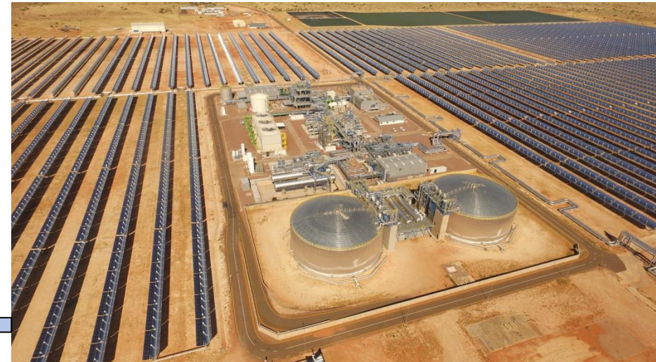
Bokpoort CSP Plant (Sener). Source: www.solarpaces.org
