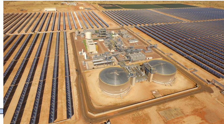
Bokpoort CSP Plant (Sener). Source: www.solarpaces.org
