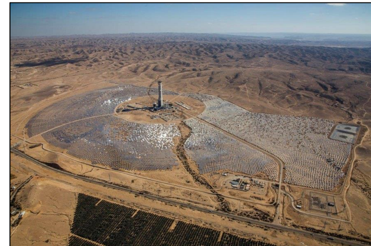
Ashalim Power Station, BrightSource Industries Israel (source: https://inhabitat.com/ )
