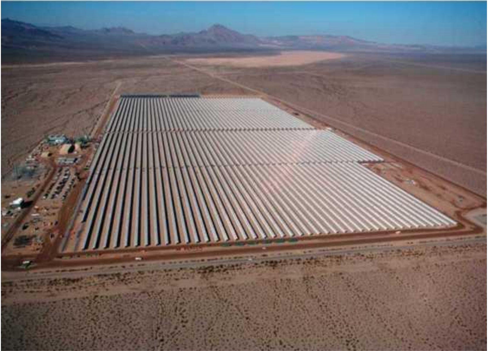
NEVADA SOLAR ONE - ACCIONA SOLAR POWER
